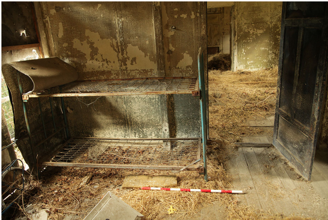
Figure 6. Initial overview of Room 1. HVF Team.
