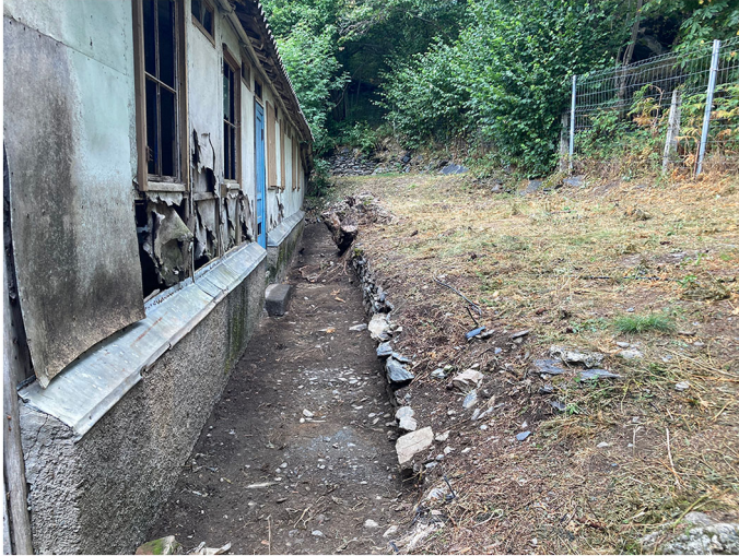
Figure 14. North area, trench excavated in July 2022. Ana Pastor.
