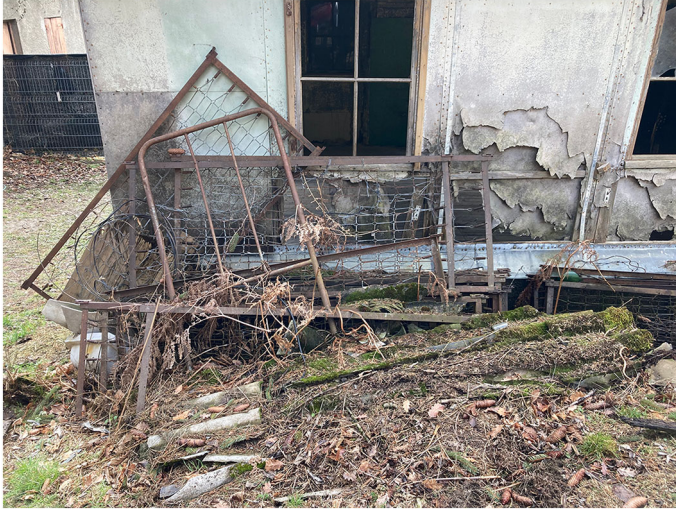
Figure 12. Accumulation of bedsteads on the north wall. HVF Team.
