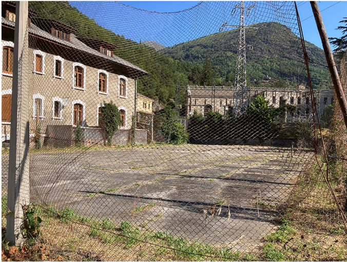
Figure 4. Cement Tennis Court in the “Poblado de la Central”. Ana Pastor.
