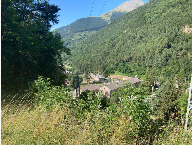
Figure 1. Capdella Hydroelectric Power Station. July 2023. Ana Pastor.
